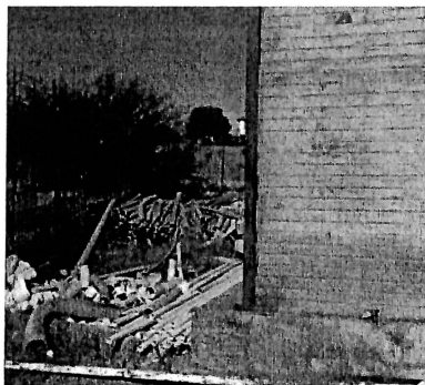
PVC pressure pipes are stored behind the garages in the sun. The pipes in the back are already sun burnt; however, they are still used for repairs for water and vacuum system.
